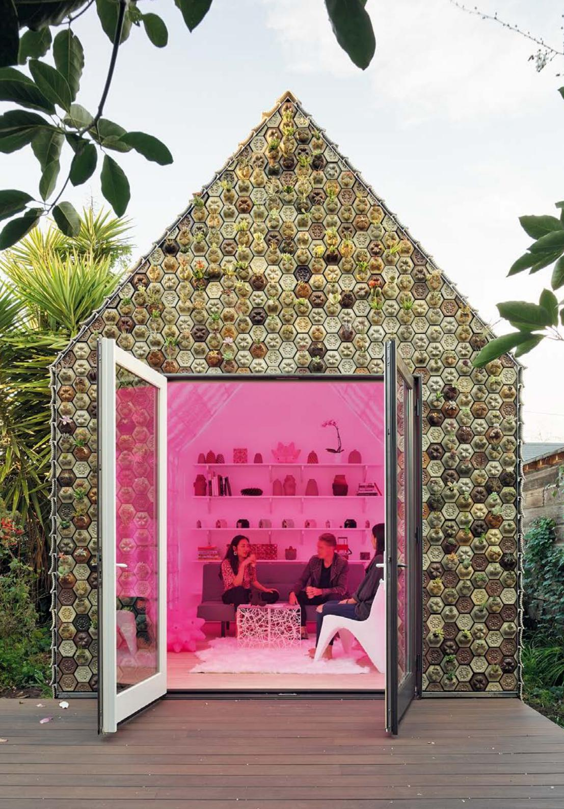
Left page: 4,500 3D-printed ceramic shingles clad the walls and roof of the cabin
