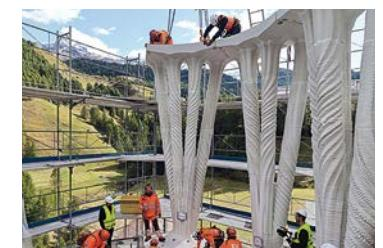
**Material:** Concrete paste extrusion, max. particle size 1.2 mm, and fast-setting
